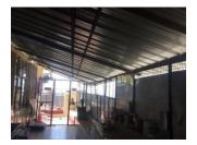
**Animal Clinic renovated:** The plastic roofing of the first aid and check up section were replaced by tin roofing. The plastic roofing has developed cracked at certain areas thereby letting in rain water whenever there is a rainfall.
